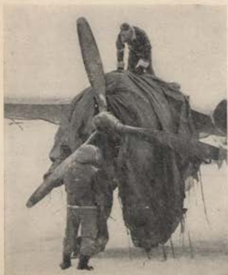
When blizzards close in the field, 100-hour inspections are performed in dispersal areas.
