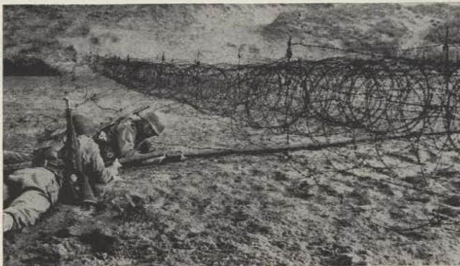
In this photograph a bangalore team has almost completed the laying of a length of pipe which will blast away the barbed wire entanglement. This method is used under conditions which make the "body-bridge" impractical.
