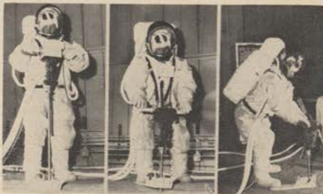
Getting to the moon is just the beginning. Tools to do useful scientific work will have to be brought along. This is one version of a lunar-surface drill, which could be used to emplace a heat probe and to get subsurface core samples.
