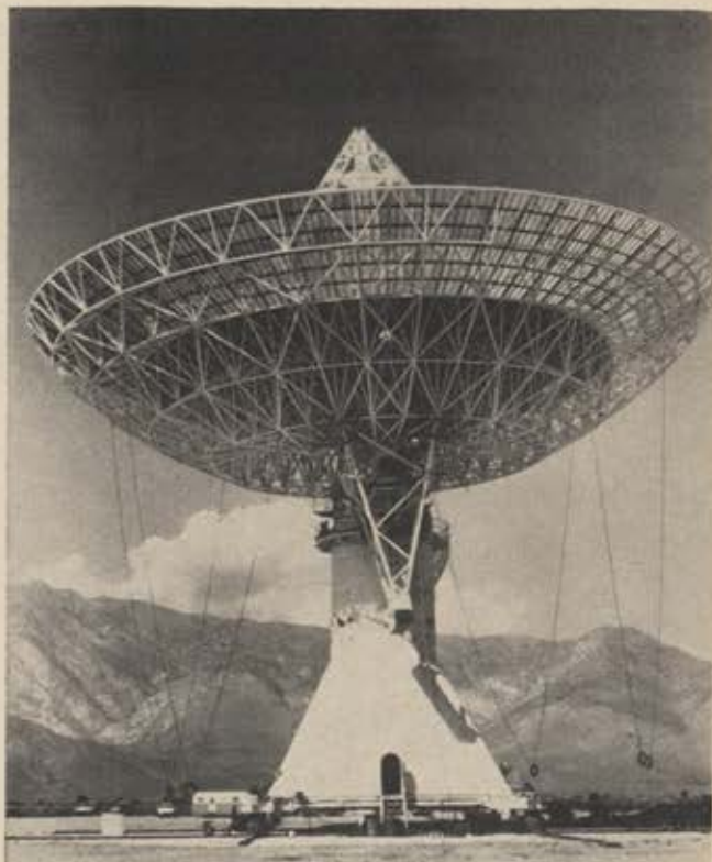
New Westinghouse-built 130-foot radio-telescope at California Institute of Technology's Owens Valley Radio Observatory, able to detect radio wave sources beyond Milky Way galaxy, has improvements over existing systems.
