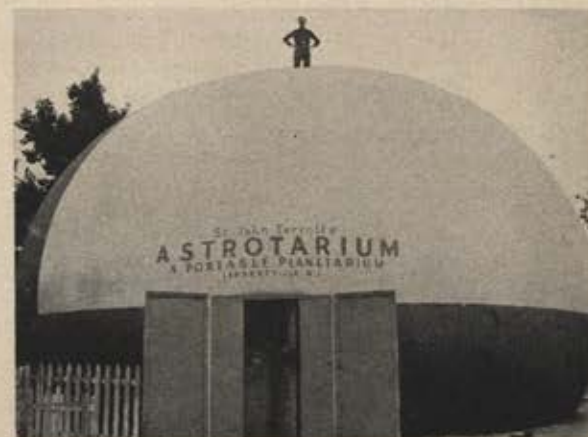
The Astrotarium, inflated nylon planetarium, is now touring the country to demonstrate the many wonders of the solar system, stars, and satellites.
