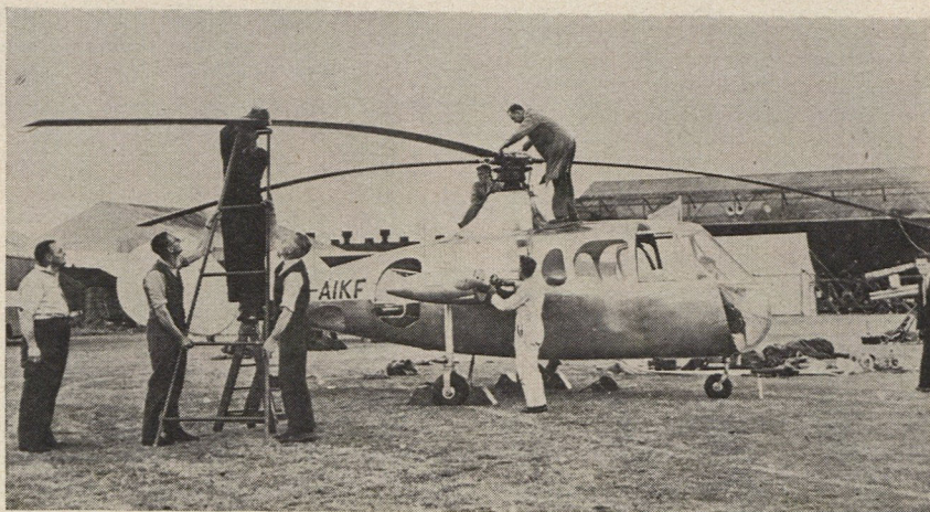
Britain's Fairey Gyrodyne is a cross between a helicopter and an autogiro. It applies power from the 525 hp Alvis engine to the rotor for take-off and hovering and to the asymmetrical propeller for cruising while the main disc autorotates.
