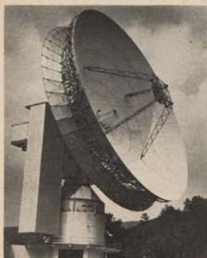
One of the world's largest movable dish antennas, located at Etam, W. Va., some eleven stories tall, was built by Philco-Ford for Comsat Corporation to provide an international communications link with satellites in orbit.
