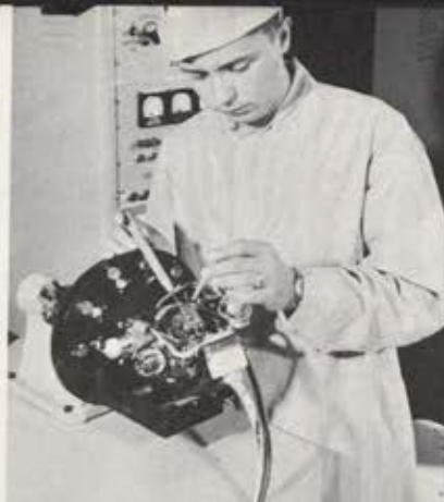
Air-bearing gyro accelerometer is tested here in Ford designed and built special fixture.
