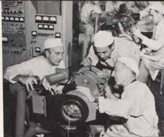
Technicians perform final checks on stable platforms for U. S. Army REDSTONE Missile in ultra-clean assembly area.
