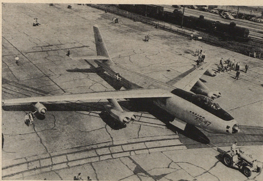
Top view of the new Boeing XB-47 Stratojet. Note how the swept-back Busemann motif is used not only in wing but also in tail and inboard engine supports. The span is 116 feet. Despite its Superfort dimensions, its crew comprises only three men.
