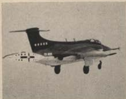
The new Blackburn NA.39 twin-jet carrier-borne strike bomber make low passes over the crowd, with tail-clapper airbrake in the open position.
