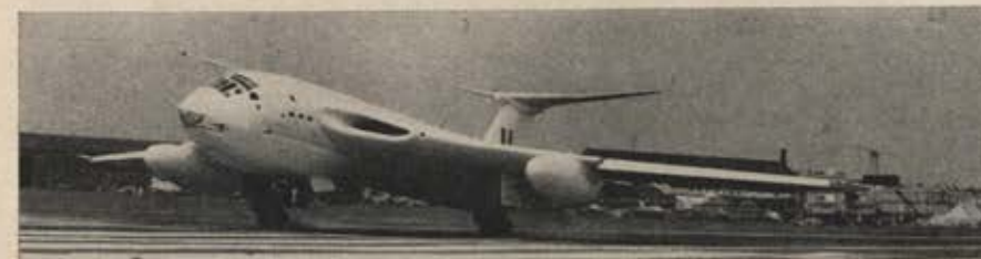
Shown with huge underwing nacelles, each housing weapons or 2,040 gallons of fuel, was Handley Page's Victor Mk. 1. The encumbered bomber flew aerobatics.
