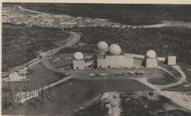
These radar domes at an installation in Canada police the air- lanes, not only detecting and tracking unidentified aircraft but guiding fighters to targets in case an air attack should ever be launched against North America. Blips on radarscopes under the domes are translated into tracks flashed on the faraway plotting board in NORAD's main Combat Operations Center.
