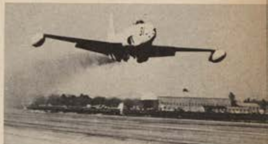
First US-built jet was the Bell P-59, powered by two 2,000-pound-thrust General Electric J31 engines. It was first flown in October 1942, piloted by Col. (later Lt. Gen.) Laurence C. Craigie. Sixty were built, but none was employed in combat.
