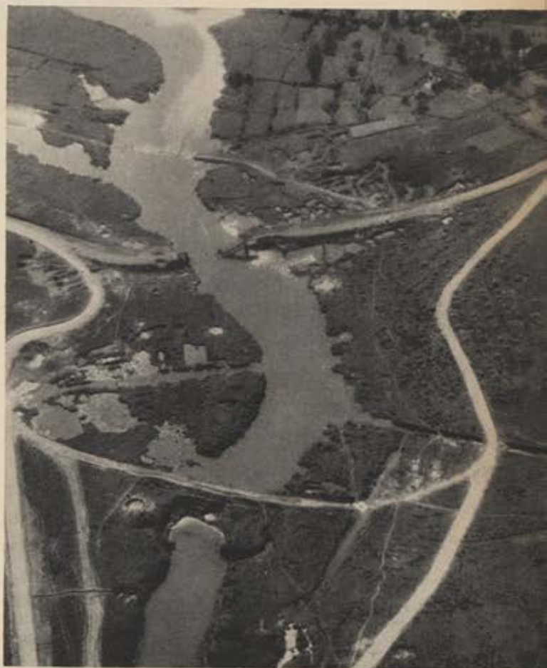
Photo reconnaissance plays an important part in campaign to interdict enemy supply routes. Repeated bombings have destroyed two bridges and cratered roads, forcing North Vietnamese to build bypass fords. Photos like these brought in by RF-101s and RF-4Cs indicate when targets should be hit again.
