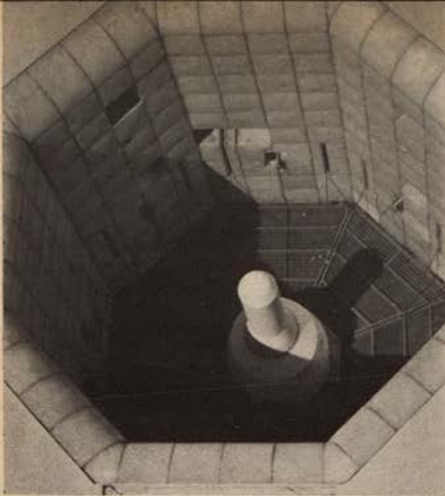
Follow-on to the Air Force Atlas ICBM was the first of the Titan series, Titan I, shown during a 1960 installation and checkout. Titan represented a major improvement over Atlas, was designed to be launched from underground silos, protected against enemy attack. Martin headed industry Titan team.
