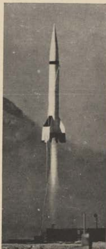
As early as 1948, development efforts were under way in the ballistic missile field. At left, a Conqair MX-744 prototype ICBM firing. Unfortunately, this Air Force-sponsored effort was cut back to save funds that were needed for the pilotless bomber program. It was only after Teapot Committee supported ballistic missile concept that we got back on the right track—concentration on ICBMs.
