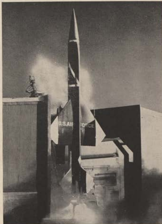
Boeing Bomarc is first SAGE-controlled intercepter missile, carries own radar to find its target 200-400 miles away.
