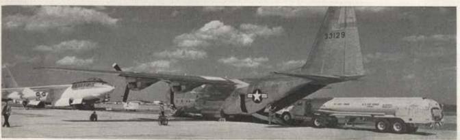
The ninety-five-foot long fuselage of the C-130A Hercules can accommodate an AF 5,000-gallon fuel tanker. Plane is designed for high, fast, long-range flights, or low and slow cargo and troop drops. The C-130 hauls a twenty-ton payload.
