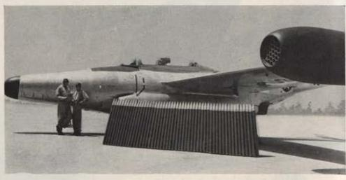
Dummy rockets in photo demonstrate the firepower carried in one of the Northrop Scorpion F-89D wing tip pods. The plane carries 104 air-to-air rockets.
