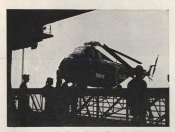
**SONAR DUNKER**—Versatility of Sikorsky helicopters is again being demonstrated in the Atlantic, where Navy HO4S helicopters now perform anti-submarine missions. By dunking or trailing special sonar gear, the HO4S is prepared to make a major contribution to the job of finding and killing enemy submarines. This HO4S, with rotor blades folded, is pictured aboard the USS Leyte.
