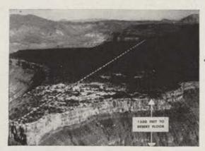
Drawing shows how new AF supersonic test sled track on Hurricane Mesa (right) will operate. Recently completed, the unit is the first of its kind built to test ejection seat equipment in free flight under controlled conditions.
