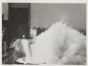
Advanced rocket engine undergoes trial at U.S. Army's Malta Test Station. The first large rocket static test station in the U.S., Malta has highly versatile facilities. Complete instrumentation gives G-E engineers extensive information on engine performance in static tests.
