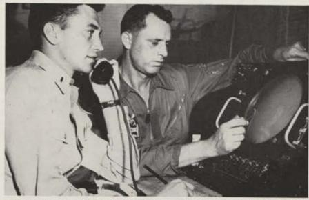
A GCI (Ground Controlled Intercept) radar controller, left, receives instruction during a proficiency rocket-firing program at Yuma. The controller gives the interceptor the speed and altitude of the target being tracked on the radar.
