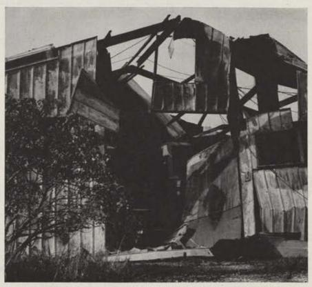
Tremendous destructive power of Typhoon Grace is well illustrated by the damage done to this Air Force warehouse on Okinawa, Winds reached 113 mph.
