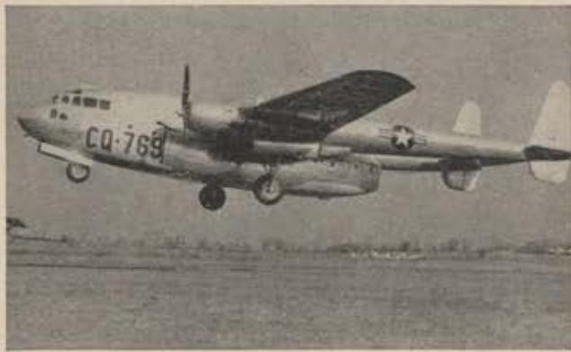
New and improved version of the Fairchild C-82 is the C-119, above, designed especially for troop carrier work in new "air transportable army." Plane has maximum payload of 31,000 lbs.
