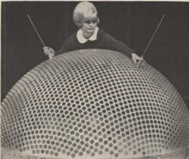
The inverted perforated dish shown above is a one-tenth scale model prototype of the advanced design array radar (ADAR) being built for USAF's Rome Air Development Center. The high-resolution ADAR under construction at Rome is designed to be a sensor for satellite identification and as a ballistic missile defense system designation/discrimination sensor. The ADAR in Rome will have a dish eighty feet in diameter and will be fitted with 16,000 rods (two are shown in the picture of the model) that will channel radio-frequency energy. The Rome ADAR is being constructed for the Air Force by Hughes Aircraft Co., Fullerton, Calif.
