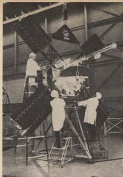
Mariner 5, shown here having its solar panel array checked by technicians before launch from Cape Kennedy, Fla., June 18, is reported working well en route to Venus flyby on October 19.
