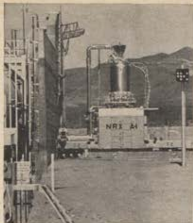
The only existing nuclear-propulsion hardware for aerospace application is for nuclear rockets. Shown here is experimental AEC-NASA test-cell installation of NERVA project, which is slated to produce about 250,000 pounds of thrust. Aerojet-General Corp. and Westinghouse Electric Co. are principal contractors.
