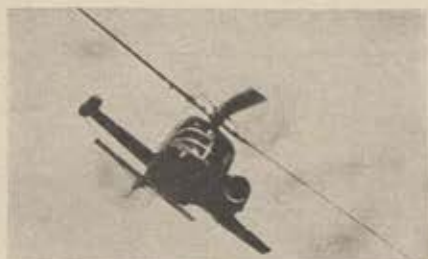
Experimental Lockheed XH-51A compound helicopter bettered its own unofficial world speed record for rotorcraft, clocking at 302 miles per hour.
