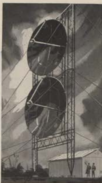
Typical 28 foot paraboloidal antennas as used in a Philco 8,000 mc forward scatter system with diversity.
