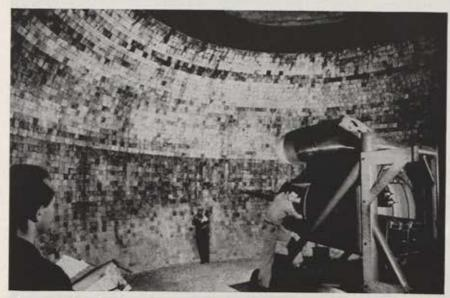
Those aren't tiles, but the ends of eight-foot timbers—over 8,000 of them. Neatly stacked, they form the inner lining of a new all-angle firing range now installed at the Evendale, Ohio, plant of the Avco Manufacturing Corp.
