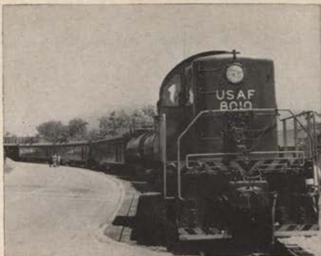
A major achievement of the original Minuteman program was development of the rail-carried mobile Minuteman system. This was what the Minuteman train looked like as it made a test run out of Hill AFB, Utah. But DoD dropped the program. The idea of mobility is being examined anew.
