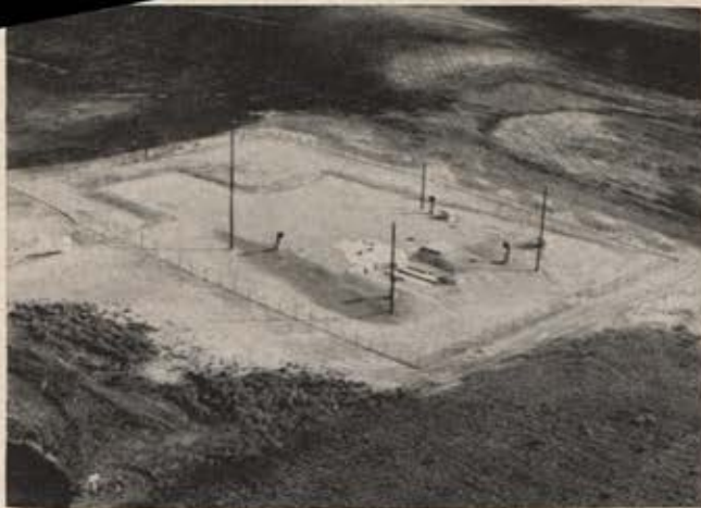
There are 1,000 Minuteman silos like this, many in midst of roaming cattle. Grass is eliminated as a fire hazard.
