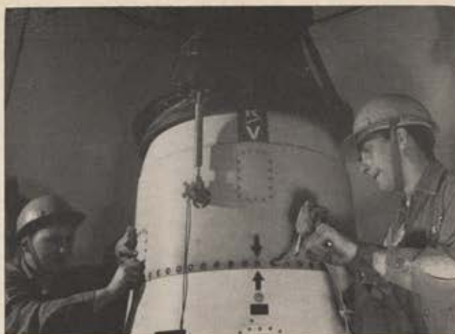
Skilled technicians are required to ready Minuteman for its vigil in silo. Installation of warhead is last step.
