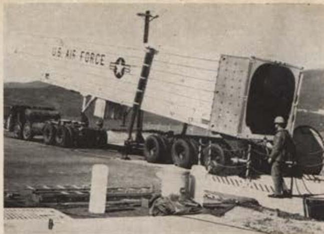
Minuteman transporter-erector is a monster truck that is capable of raising the missile and lowering it into silo.
