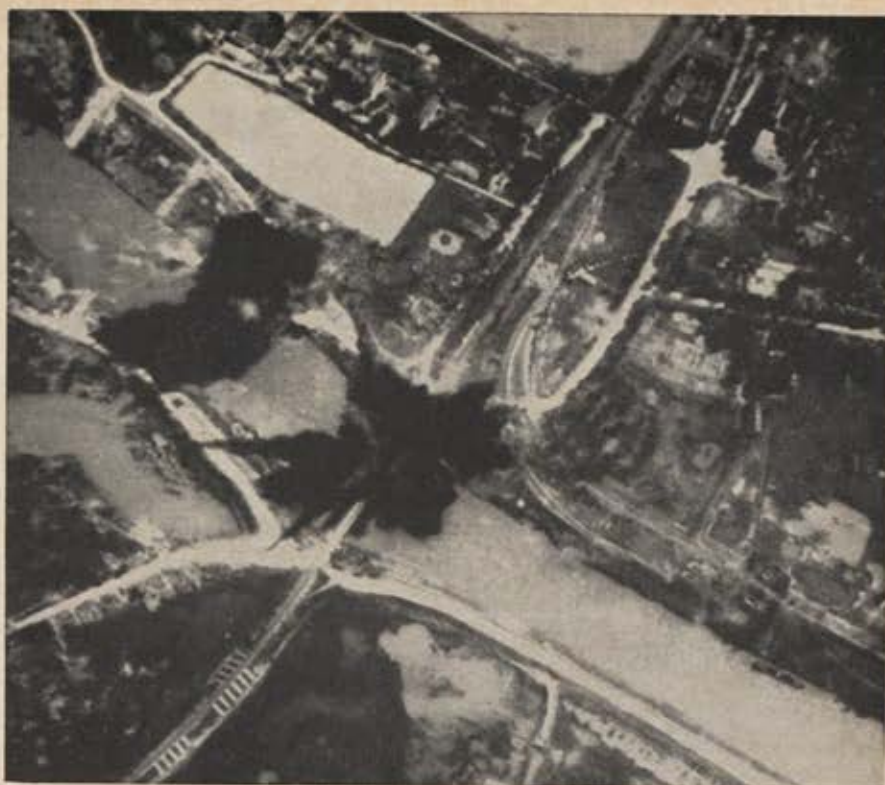
Direct hit is scored on railway bridge spanning Song Cau River at Bac Giang, thirty miles northeast of Hanoi, by 3,000-pound bomb dropped from the F-105 Thunderchief of Lt. Col. James L. Hughes of Santa Fe, N. M., member of USAF's 469th Tactical Fighter Squadron based at Korat, Thailand. Rail line snapped by Colonel Hughes is one of two main arteries serving Hanoi from Red China.
