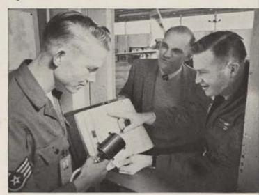
4. NEW CDP SENSOR, picked up at the Squadron's spare parts stock room, will be installed to complete engine minor repair, ready J47 for reinstallation . . .
