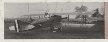
The final version of the Spad was the model 16, a two-seat fighter that first appeared in June 1918.
