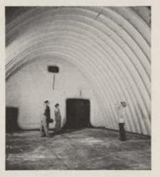
Inflated rubber air columns form roof and walls of new AF aretic shelter.
