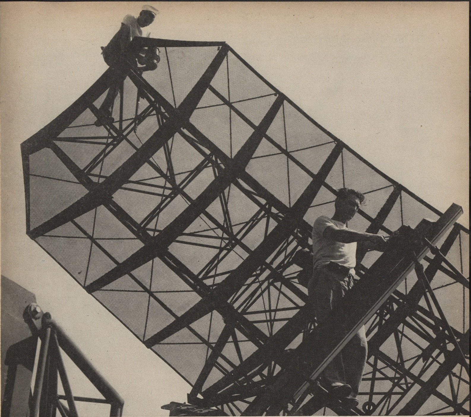
To furnish weather data for Thunderstormers, the Weather Bureau has set up a network of 63 stations in Clinton area. Above, a section of the giant V-Beam capable of covering 200 mile radius.
