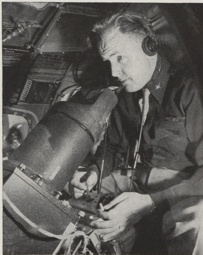
Television Scope in nose of Mother plane records what is happening to instruments in Babe plane. By watching scope Capt. J. A. Evans, a beeper pilot, flies Babe plane with special control stick box.
