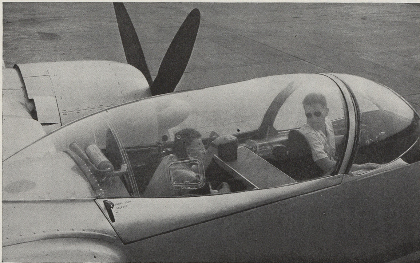
This giant transparent "bubble" which forms a smooth and streamlined section of the fuselage affords F-15 pilot 360 degree vision.
