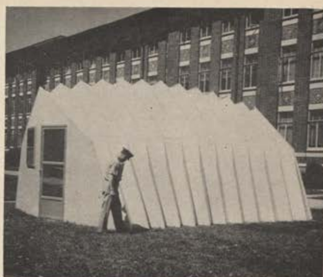
Tactical Air Command is preparing a new concept that will permit fast deployment to "bare base," equipped in advance only with runway and water. This is a collapsible shelter.
