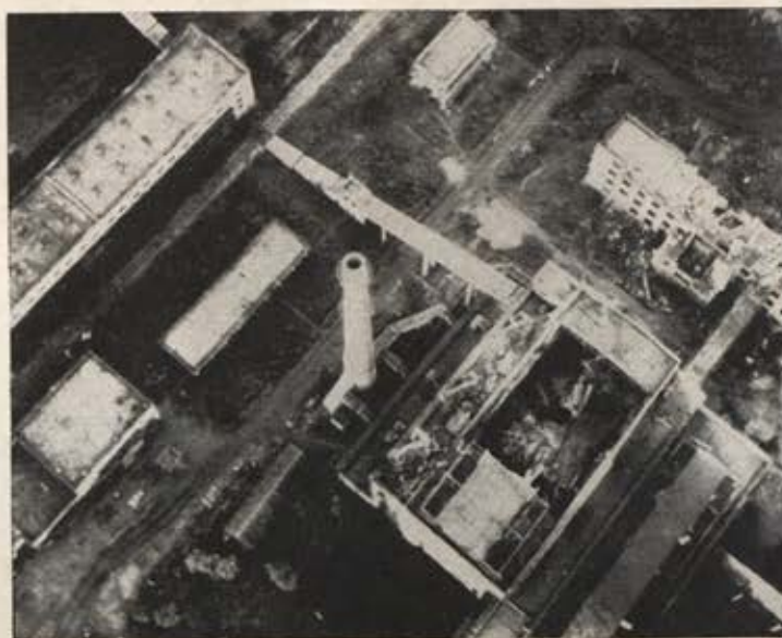
Recon photos as above are often used for damage assessment. Here massive damage done to Thai Nguyen thermal powerplant, located thirty-eight miles north of Hanoi, is shown. The plant supplied seventeen percent of North Vietnam’s electrical power before the F-105s clobbered it.
