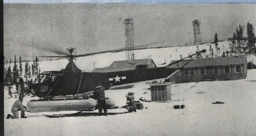
The first Arctic helicopter rescue was made with this craft. Here GIs place a canvas mat under the helicopter as it settles, to keep pontoons from freezing.
