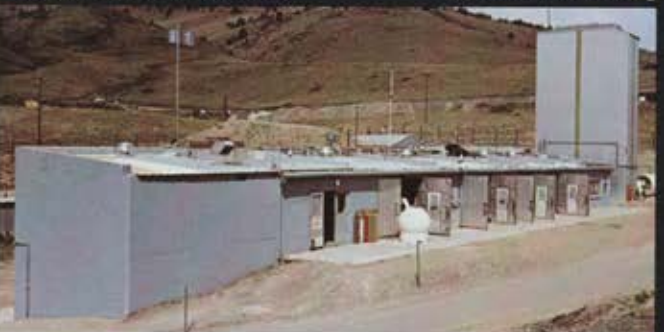
Boulder... Hazardous Testing
