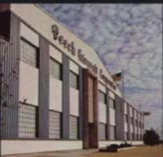
Wichita, Kansas, Plant II
