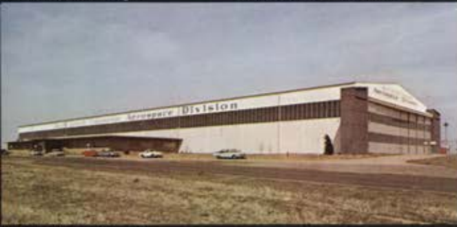
Wichita, Kansas, Plant III
