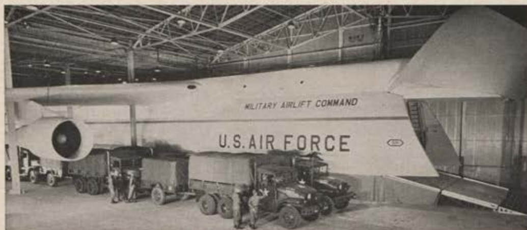
C-5's ability to carry a 265,000-pound payload, including outsized, bulky items, is portrayed by mockup showing the nineteen-foot-wide cargo compartment. Double row of six trucks and trailers can be accommodated with space for center and side aisles.
