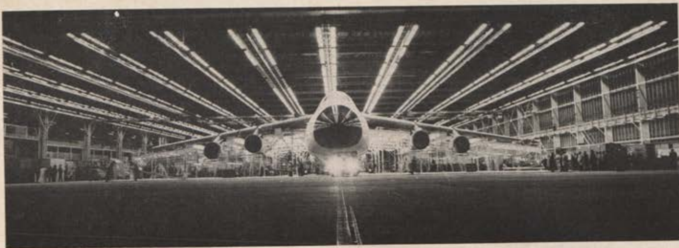
First prerollout "outing" of C-5 took place when aircraft number one left main manufacturing building for empennage-mating hangar—a specially designed structure at Lockheed-Georgia plant where C-5 fuselage was mated with 65-foot-tall tail.
