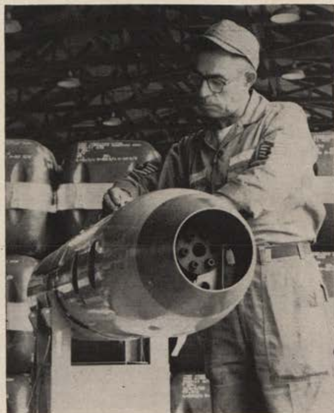
A weapon of major importance in the effort to produce a high level of sustained firepower in order to hold off guerillas during surprise attacks is the six-barrel, 6,000-round-per-minute Minigun used on many aircraft in Vietnam.
