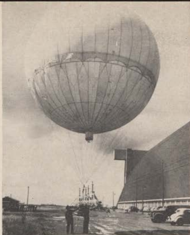
A captured Japanese balloon, inflated under test conditions, shows scallop to which shroud lines were attached.
