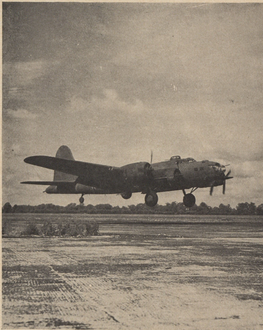
The only visible difference between the B-17F, shown above, and its predecessor, the E, was elongated plexiglas nose, which allowed bombardier more vision and room.
