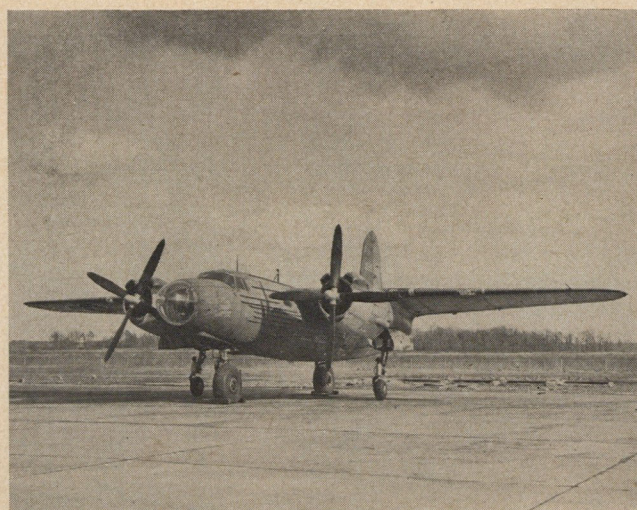
Army authorities are still secretive about benefits to be derived from this unusual landing gear setup experimentally installed in the Martin XB-26H. The tandem fuselage wheels are the same size while balancing wheels in nacelles are considerably smaller.
