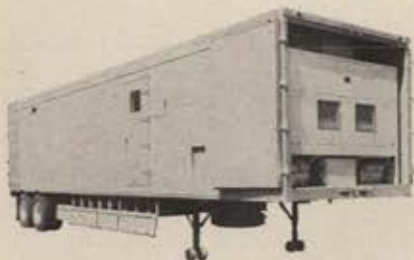
ONE OF THREE DORSEY UNITS that make up the transportable COMSAT Earth Station designed by Northrop Page Communications.
