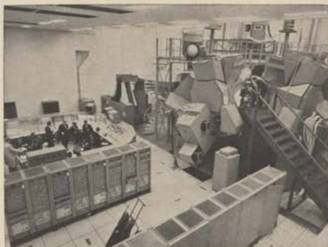
It looks for all the world like a space-age jungle gym that kids would go wild in, but it is the MSC Apollo Mission Simulator, one of the principal astronaut training facilities crucial to preparation for the real thing—coming soon.
