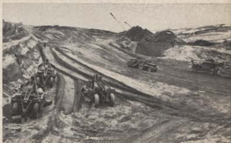
American troops landed on Amchitka in January 1943. A month later fighters were operating from the new airstrip, and by March medium and heavy bombers were striking Kiska. Here trucks haul sand for runway foundations.
