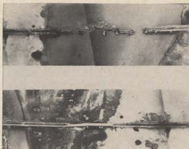
Putting a bridge out of commission is one thing; keeping it that way another. Composite photo shows destruction of eastern portion of bridge near Hanoi by USAF F-105s in December (top). Western section of same bridge, damaged last October, has been almost completely rebuilt (bottom).
