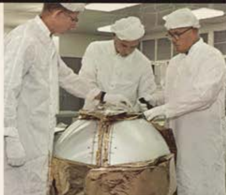
The design and fabrication of pressure vessels and cryogenic storage systems are highly developed at Beech. This cryogenic storage system was designed and built by Beech under contract with North American. It was the first of 13 major subsystems aboard the Apollo spacecraft to be man-rated by NASA.
