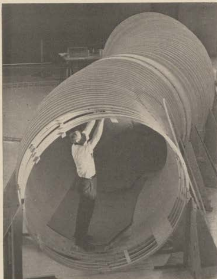
Full-scale mockup of the world's largest inlet duct for an aircraft engine takes shape at Lockheed-California's Burbank facility. The "S-duct" will channel air to the No. 2 engine of Lockheed's L-1011 advanced trijet aircraft. This duct is to go into a full-scale mockup of the L-1011.
