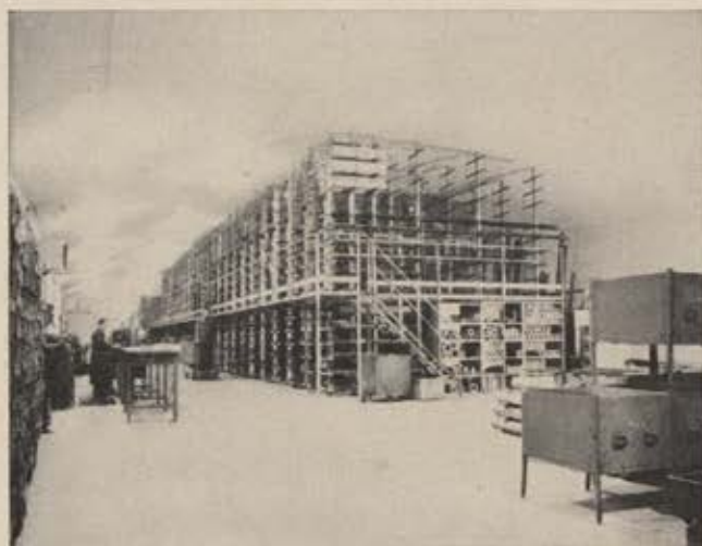
After Hiroshima, Sweden began building underground factories. This is a SAAB Aircraft Co. parts and tool room.
