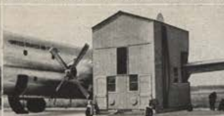
STANDARDIZED MAINTENANCE SHELTER for heavy aircraft. Portable, enclosed, weather-proof.
