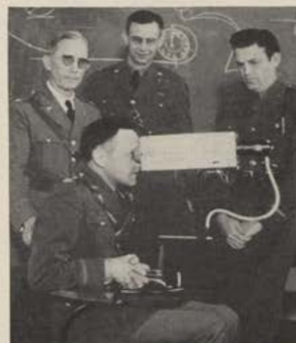
An Ocker device used in blind flying instruction at Randolph Field, Tex.
