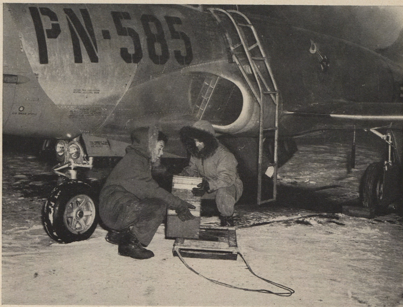
Shooting Star crew installs batteries prior to take-off. Planes were modified to start on gas.
