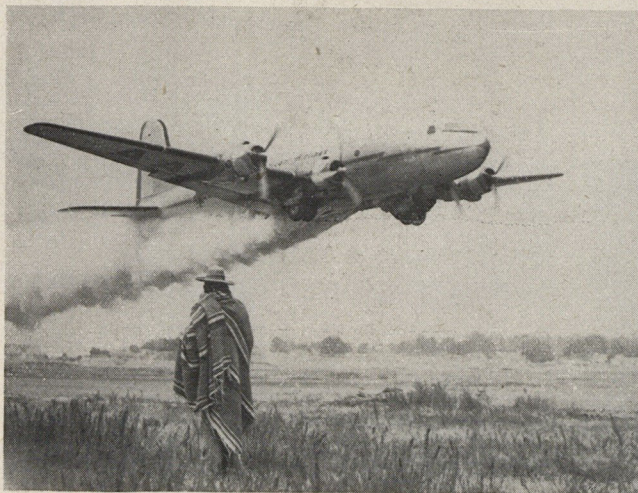
Mexican native watches American Airlines freighter taking off with a record load from Mexico City using JATO (Jet Assisted Take Off).
