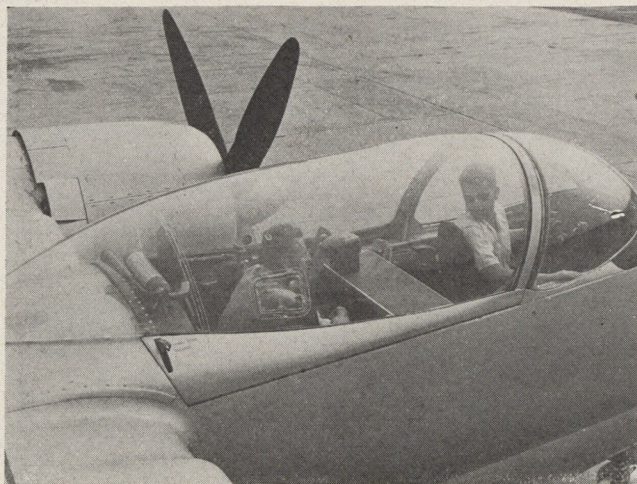
Postwar plane procurement by the AAF included the F-15 Northrop Reporter, an alteration of the famed P-61 Black Widow. Changes were chiefly in the main nacelle, with guns and radar eliminated.
