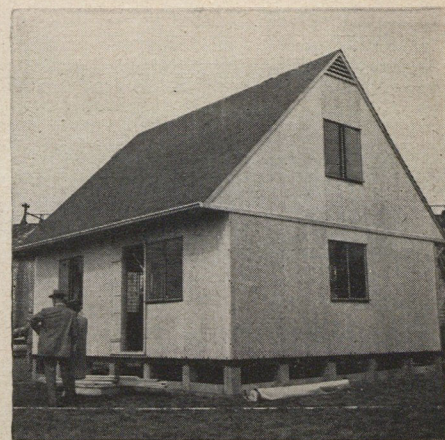
5 Small crew enclosed house, 20 by 24 ft., in a day. No part weighs over 75 pounds.
