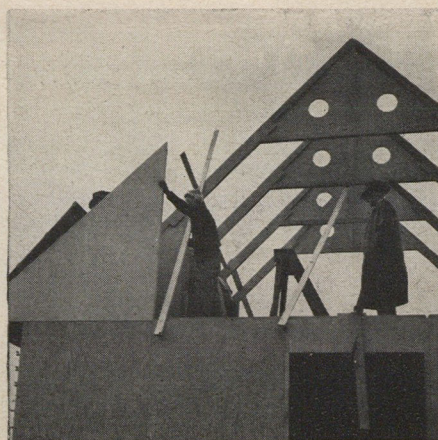
4 Roof frames of built-up plywood have integral bracing, are notched for decking.
