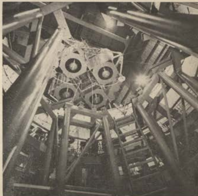
Wyle Laboratories, El Segundo, Calif., test-assembled Saturn V's major stages for Apollo in a record four months at Huntsville, Ala. Above, mated LM is hoisted for assembly.
