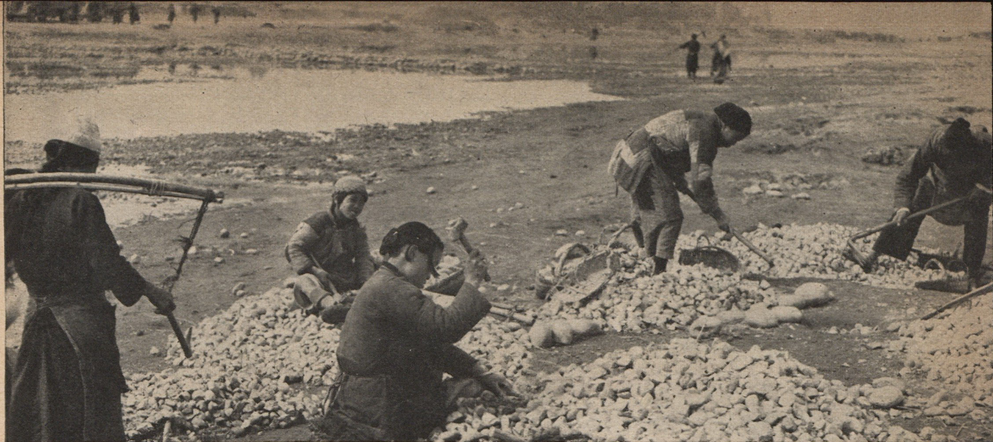
Airports grew up all over the world. Here a group of native workers in China smash rock in making a landing strip for B-29s.
