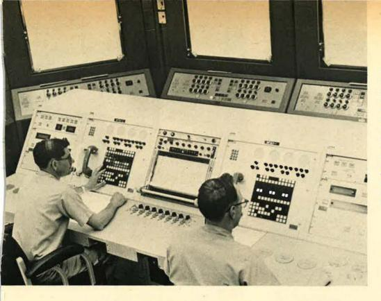
During a launch, the Missile Flight Safety Officer sits at a console, facing a series of Plot Boards that show the missile's position and predict where it would land in case of a "destruct" command or a malfunction. The MFSO also receives data from ground observers and telemetry from the missile itself. The missile is never allowed to stray from its assigned safety corridor.
