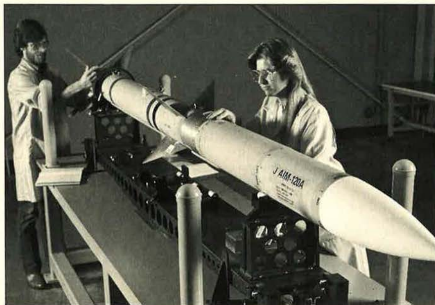
The 128th and final missile in the Advanced Medium-Range Air-to-Air Missile full-scale development effort is prepared for weight and balance testing at the Hughes facility in Tucson, Ariz. First deliveries of production AIM-120s will begin this month. Raytheon is the second-source manufacturer for AMRAAM.
