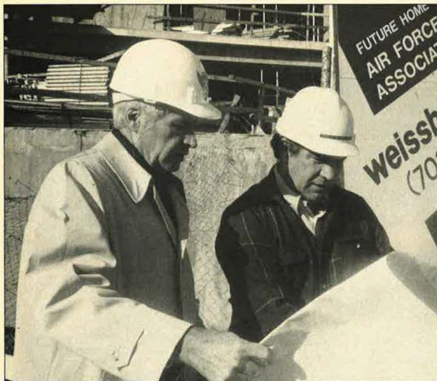
AFA Deputy Executive Director Andrew B. Anderson, left, who has directed AFA's new headquarters building project since its inception, reviews a blueprint with construction superintendent Ernie Blankenship. (Photo by Ken Goss)
