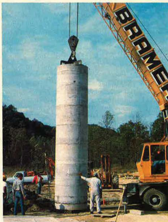
A one-eighth-scale model of a superhard silo is lowered into a pit at Fort Polk, La., in preparation for an explosive test. The silo, made of steel and concrete, is more than ten times harder than previous US silo designs tested in the past decade.
