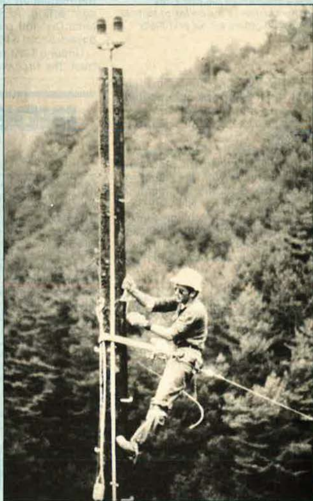
Sgt. Robert Foley installing a high frequency antenna during construction of the Korean Tactical Range, KOTAR. (USAF photo by TSgt. Bertram W. I. Mau)
