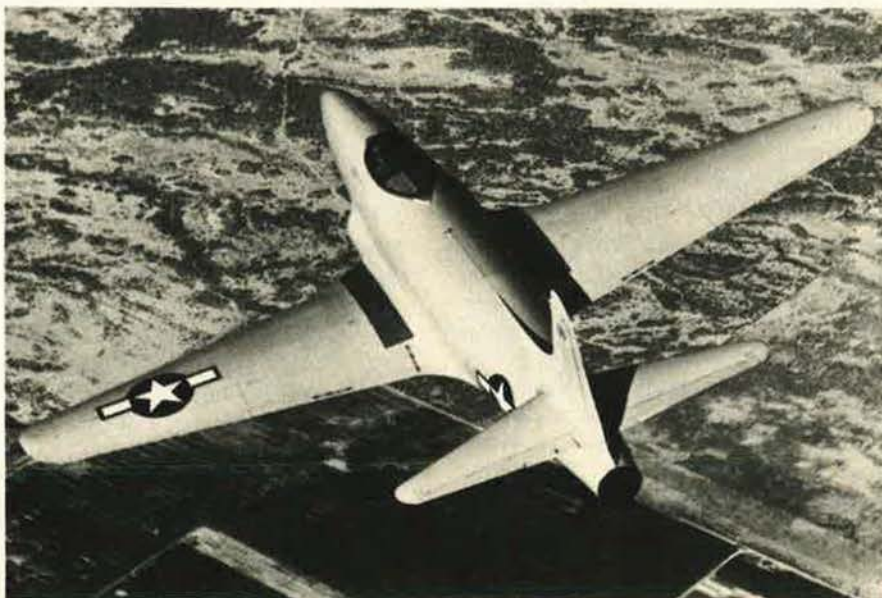
The first American production jet fighter was the Lockheed P-80 Shooting Star. Powered by GE I-40 engines with 3,750 pounds of thrust, the P-80 still proved almost 100 mph slower than the Gloster Meteor. (USAF photo)
