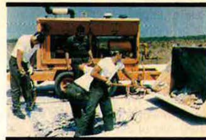
LEFT: F-15 cockpit instrument display. Far greater range of information is provided to the pilot without increasing panel size or number of instruments to monitor. Much of the information is projected on a HUD, so the pilot's attention can remain outside the cockpit. ABOVE: Air Force personnel removing buckled concrete from edge of small explosive crater. Craters from an airfield attack may range up to sixty feet in diameter. BELOW LEFT: Gen. Robert T. Marsh, AFSC Commander. BELOW: Ground crew member installing an electrical component in an F-15.
