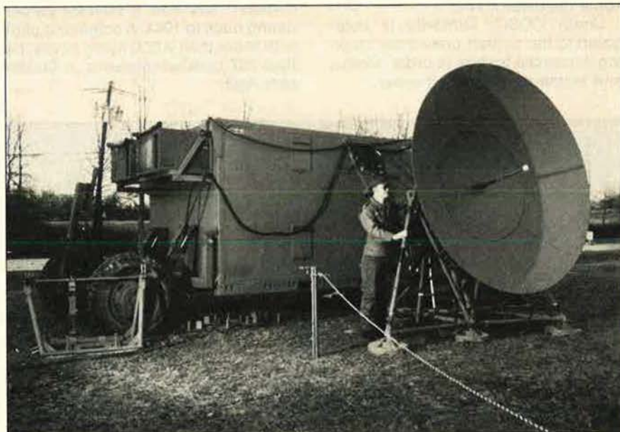
The antenna of the US Army's new AN/TSC-86 terminal is aimed at a communications satellite in a test program at RCA facilities in Cherry Hill, N. J. The strategic and transportable ground system is the first of six designed to provide instant communications among Army commanders located in close proximity or half-way around the globe.
