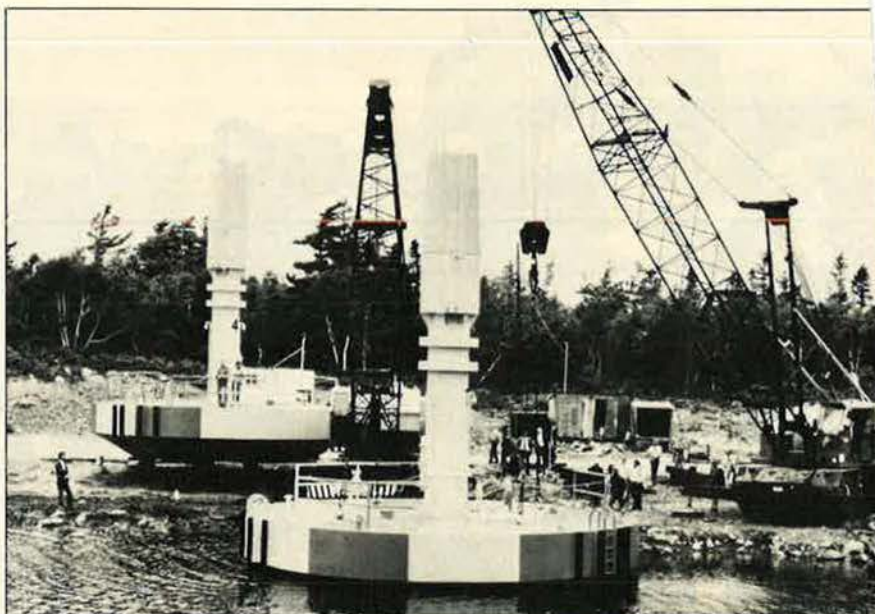
Four buoys like the thirty-five-ton behemoths shown above are to provide the cornerstones of a computerized dogfight training system encompassing 700 square miles off the coast of Sardinia, Italy. The three-dimensional system, built by Cubic Corp. and known as the Air Combat Maneuvering Range/Instrumentation, will be used to test the skills of US Navy and USAF fighter pilots and those of our allies. The range will be operational this summer.
