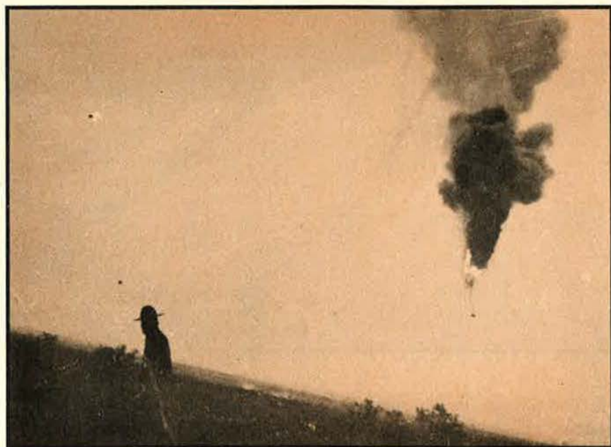
Disaster, as an Army balloon comes to a flaming end near Ft. Sill, Okla., in the summer of 1935. Static electricity, the product of nearby rain showers, was believed to have ignited the highly flammable hydrogen lifting agent.
