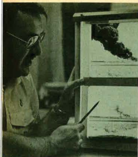
Maj. Donald Silva shows how a water-injection system reduces smoke from burning fuel during fire-fighting practice.
