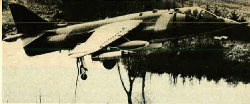
The British-built Harrier V/STOL, or AV-8A as it is known to the US Marine Corps, is limited to an 8,000-pound payload on vertical takeoff.
