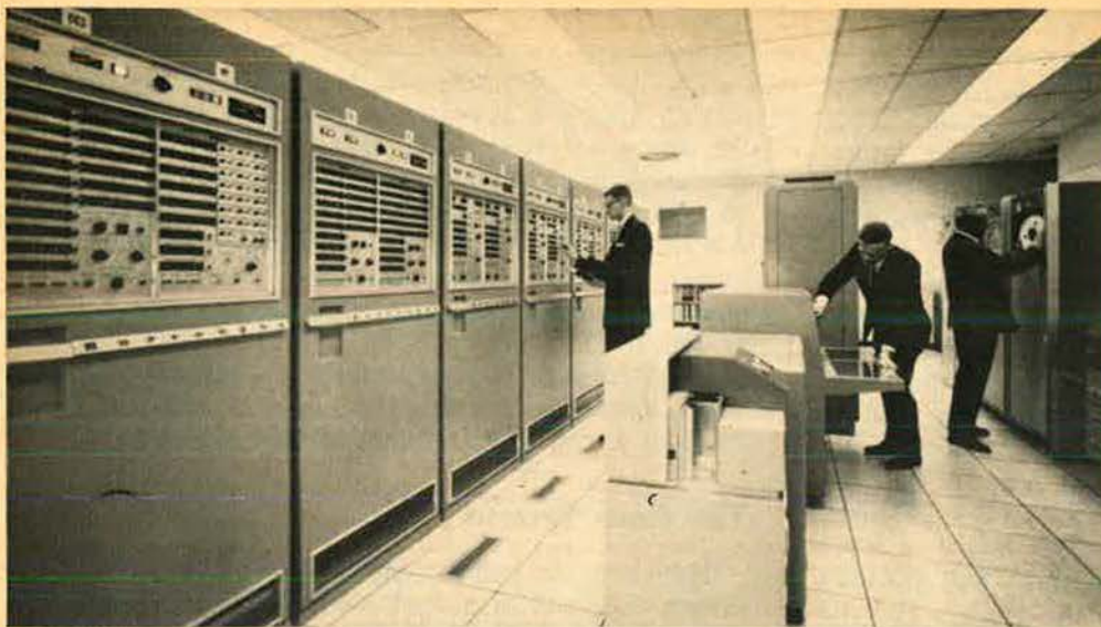
Burroughs D825 Data Processing System is core of the present, ground-based Backup Interceptor Control (BUIC) system which performs part of the continental air defense mission. Present CONUS air defense system relies on fixed ground-based radars and control centers of SAGE, BUIC, and a limited force of EC-121s equipped as radar picket aircraft.
