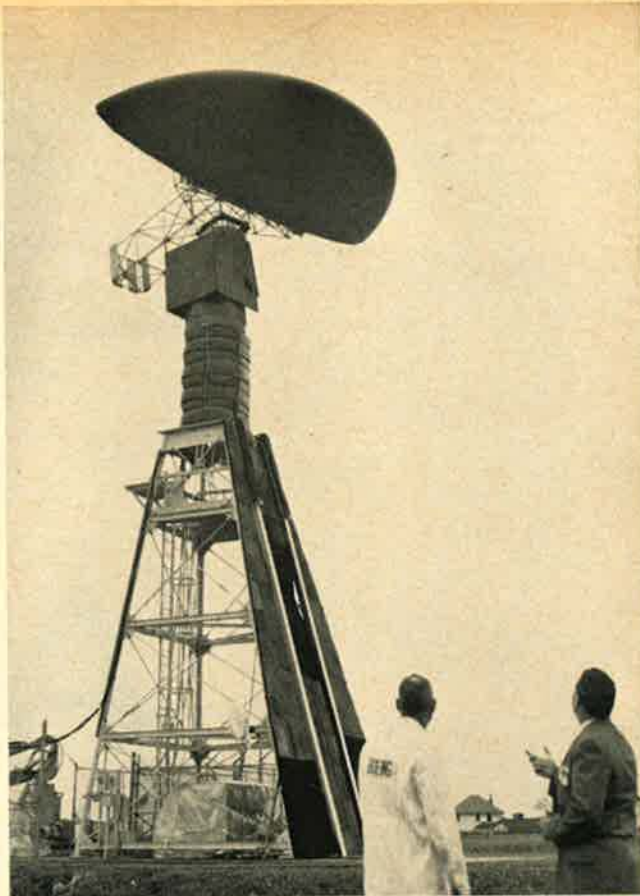
At the Boeing Space Center, Kent, Wash., an AWACS radar antenna, probably the largest ever built in a single piece, rotates atop a sixty-five-foot tower in test runs.
