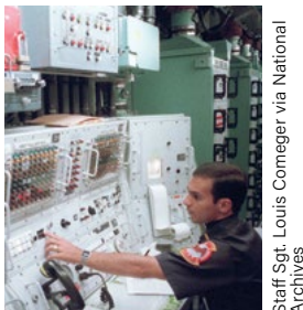
A member of the 321st Strategic Missile Wing, Grand Forks Air Force Base, N.D., at a control panel inside a Minuteman III ICBM silo, June 15, 1983.
