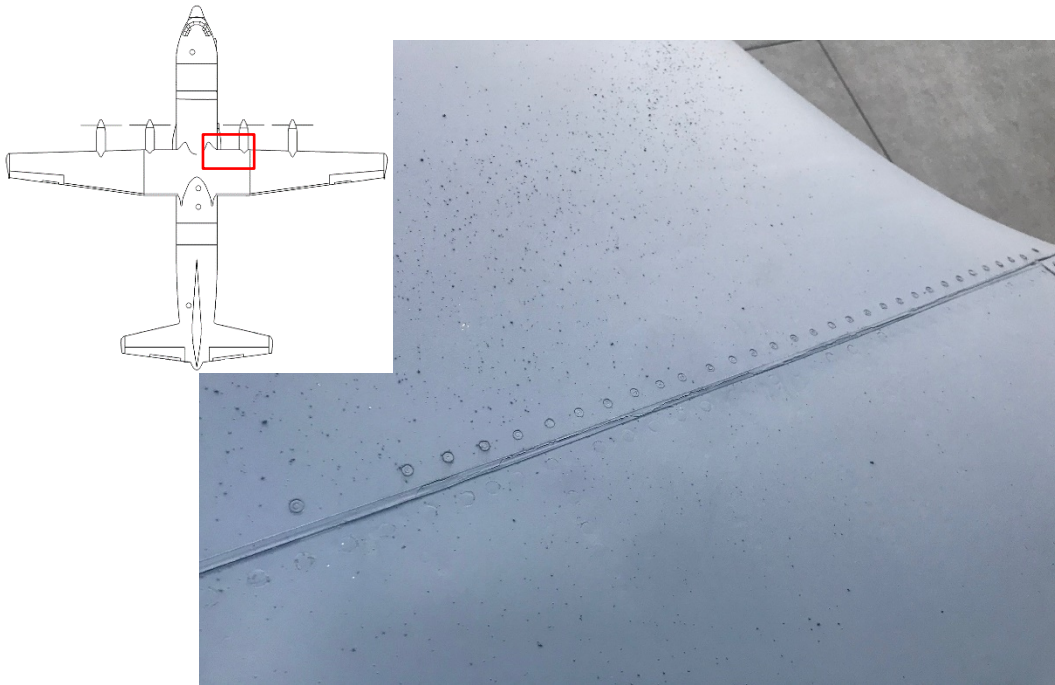
Figure 26: Right Hand Forward Wing Box at FS517, Pulled Rivets (aircraft aft to forward perspective) (Tab S-18)
