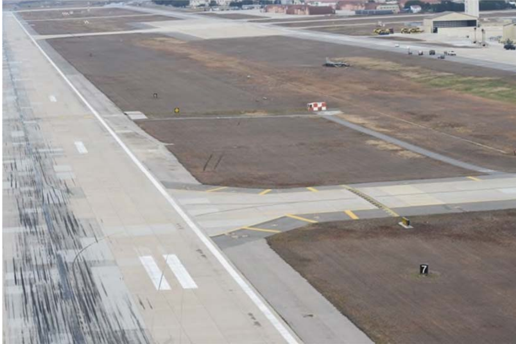
Image 15. Mishap Site Looking North; Runway Witness Marks Leading Into the Grass (Tab Z-7)
